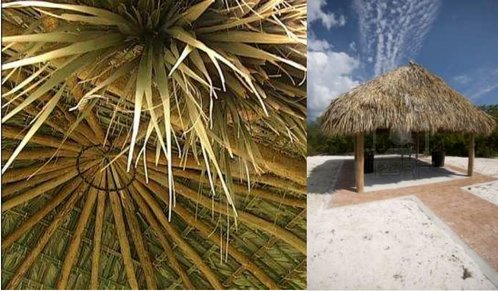
Figure 3.1.: examples of thatched roof structures ( http://www.123rf.com/photo_2683641_thatched-roof-tiki-hut-shelter-in-florida-keys-beach-entry-marathon.html ).
